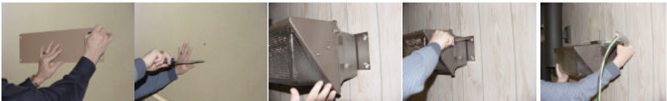
STEP 1. Mark wall with supplied template.
